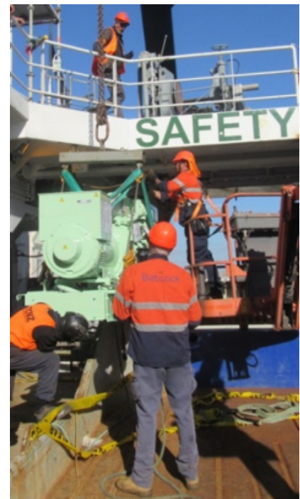
Tangaroa - Replacement harbour generator
